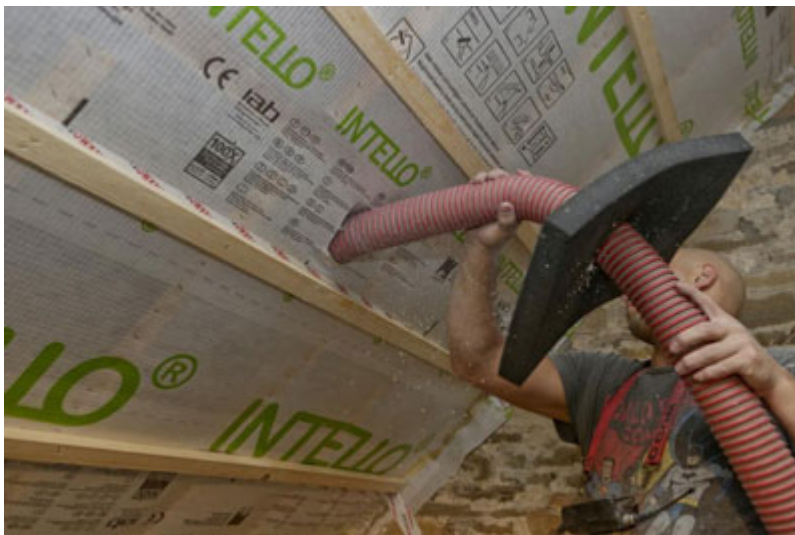
Insufflation de cellulose. Photo : Ecobati .
